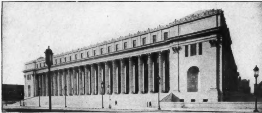
UNITED STATES POST OFFICE, NEW YORK McKim, Mead & White, architects, New York. S. Homer Woodbridge, engineer heating and ventilation, Boston
